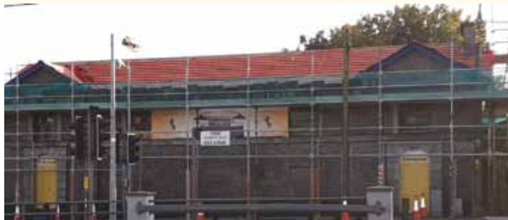
Scaffolding erected, slates removed, roof damage repaired, felt underlay installed awaiting slaters to affix the old slates
