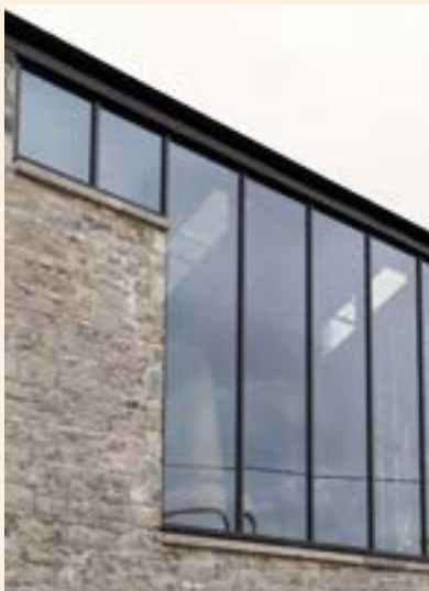
Renovated exterior of Ahascragh Distillery with Copper Stills pictured inside
